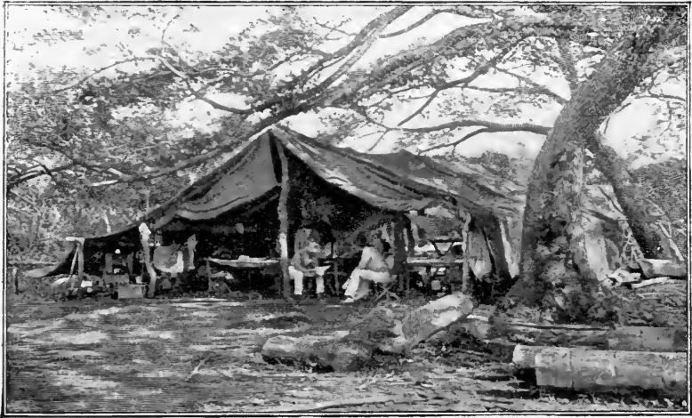
Engineer Camp of the Nicaragua Railway on the West Side
